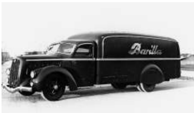
Left, the streamlined Fiat 635 RNL van (1937) [Archivio Storico Fiat, Turin] with bodywork by Viberti on a bus chassis and 6-cylinder, 8355cc engine. Below, it was used in a commercial brochure due to its refinement and elegance [Archivio Storico Viberti, Turin].
